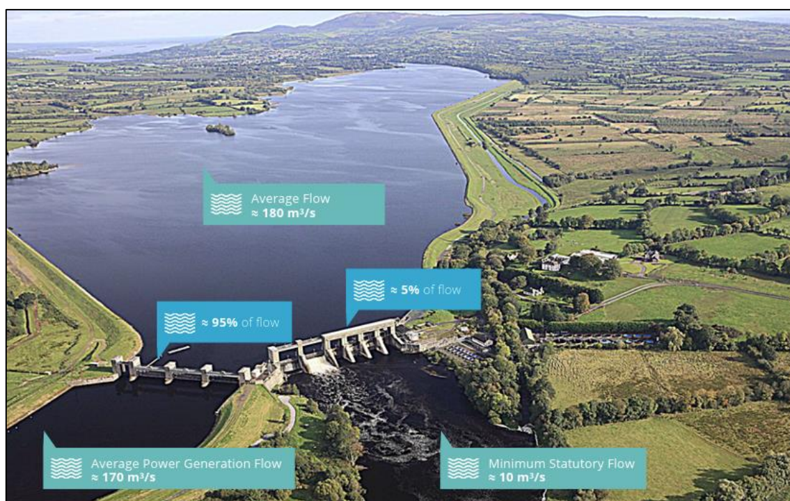
Figure 7.1 – Annotated Photograph of Parteen Basin (Source: Uisce Éireann)
